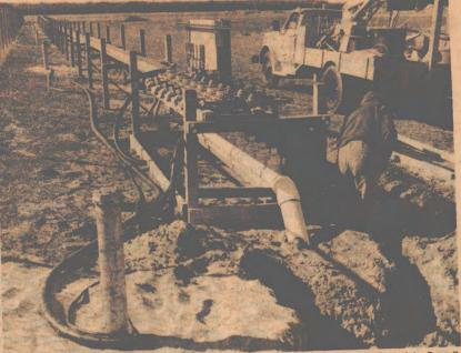
Wells lining the eastern fence of Coast Guard Air Station property will be used starting Friday to stop the flow of contaminated water off of government property. The polluted water will be pumped to four large activated carbon filters which will remove contaminants.
