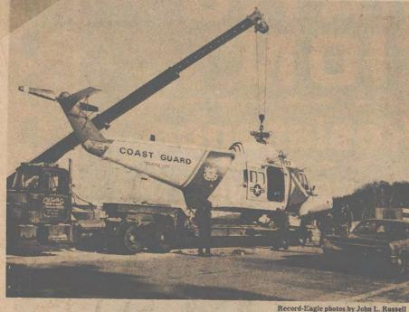
A crane lifts the helicopter onto a flatbed truck.
