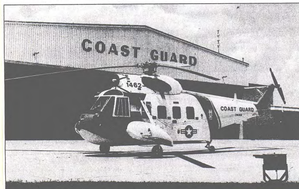
The United States Coast Guard facility was located to the north on the air station property. A new hangar provided space for helicopter storage as well as room for aircraft maintenance and administrative offices.
